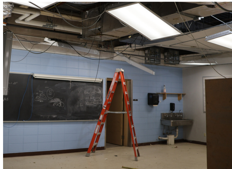
Amery High School Art room demolition
